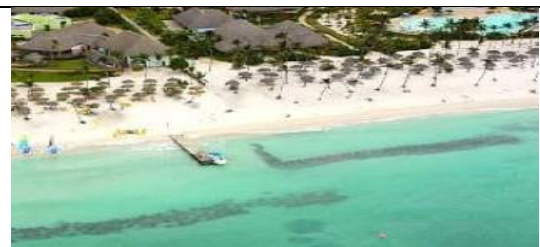
Figure 5 Picture of submerged breakwaters
