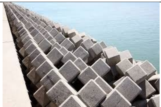
Figure 2 Breakwater with concrete shaped blocks
