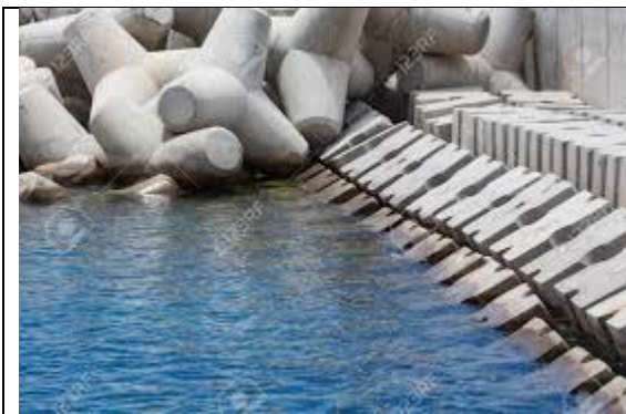
Figure 1 Breakwater with concrete shaped blocks
